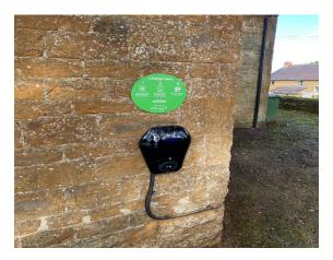
The new EV charger is sited on the side wall of the hall. It can be accessed by downloading the EV charge Online App – the detailed instructions are mounted on the wall above the unit.
